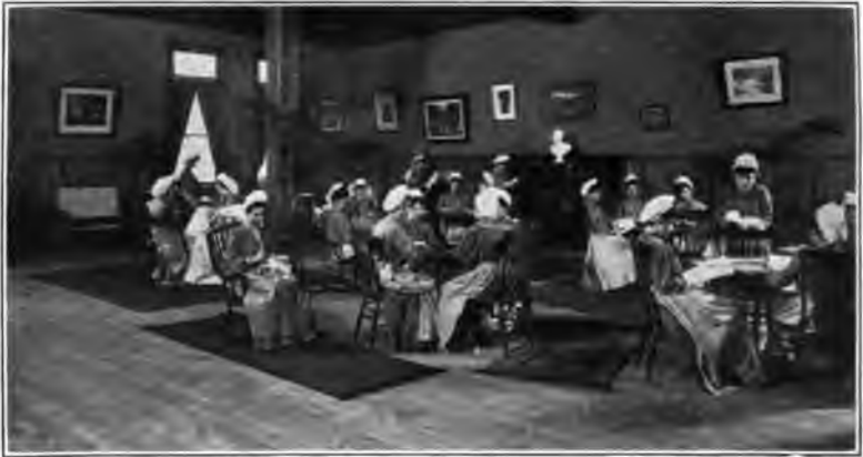
RECREATION ROOM FOR EMPLOYEES
